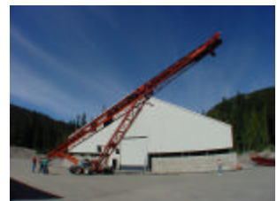
This shed stores sand for maintaining safe conditions on icy roads.
